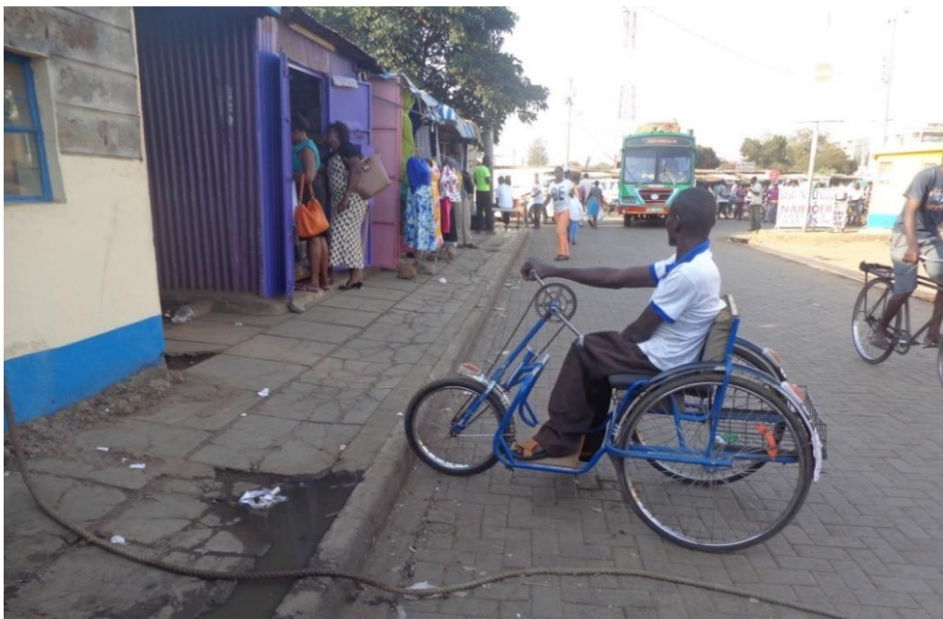
Plate 4.3: Tricycle User unable to Access Pavement due to High Kerb (Kisumu Bus Terminus). Source: Field Data, 2015
