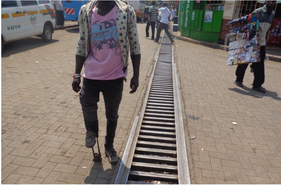
Plate.4.5: Wide Drainage Gratings Present a Mobility Barrier.to Special Boot User
