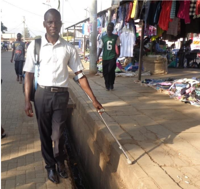
Plate 4.4: Open Drain Along Pedestrian Pathway- Kisumu Terminus
