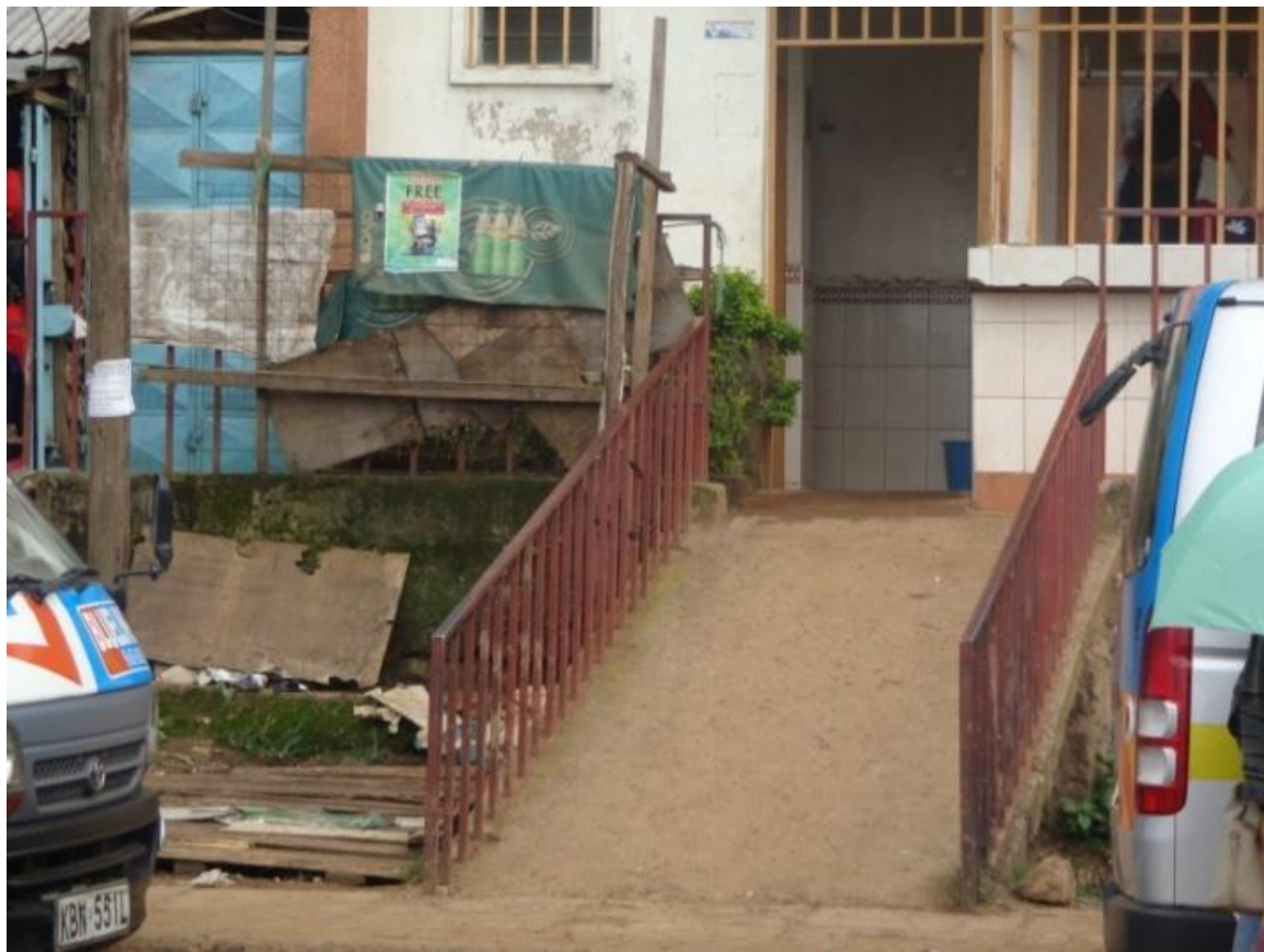
Plate 4.15: Ramped Walkway at Washroom Entrance (Kakamega Terminus)
