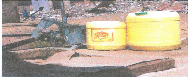
Plate 1: Semi open water well, fixed with pump but sited near pit latrine (arrowed) and solid waste dumpsite in Nyalenda "B" informal settlement. Source: Field photography.
