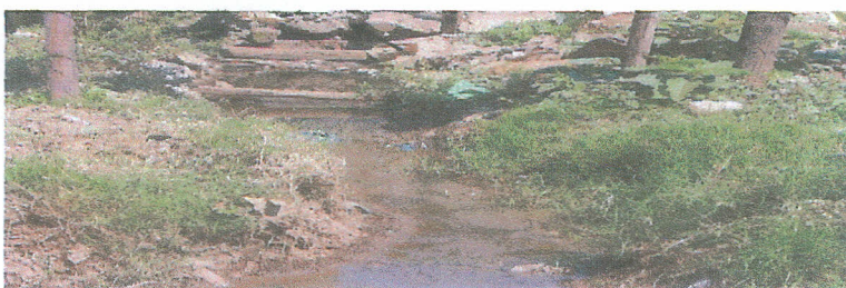
Plate3:Over flowing pit latrine (arrowed) in Nyalenda "A" informal settlement. Source: Field photography.
